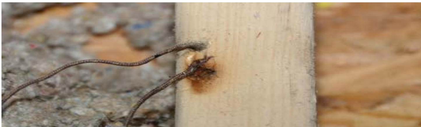
Figure 9 – Photograph of thermal damage to the wood around the screw head taken after the end of the first test.
