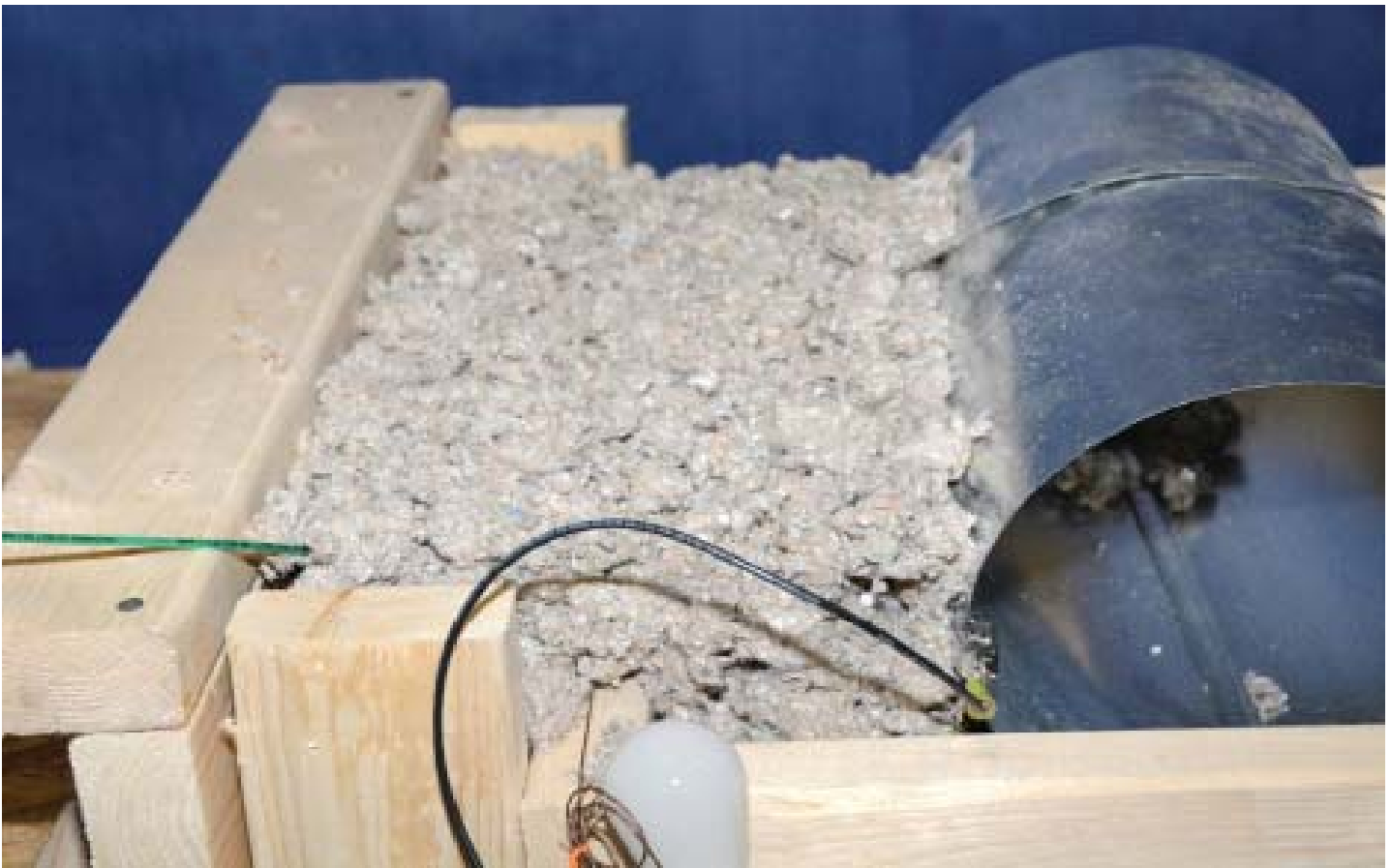
Figure 4 – Photographs of the Energized Duct / Grounded J-box test setup showing the connections between the metal strapping, screw, and J-box (top) and the setup after addition of the cellulose insulation (bottom).
